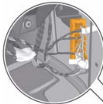
Junction boxes 2 and 3 for bus systems, on the right A pillar
